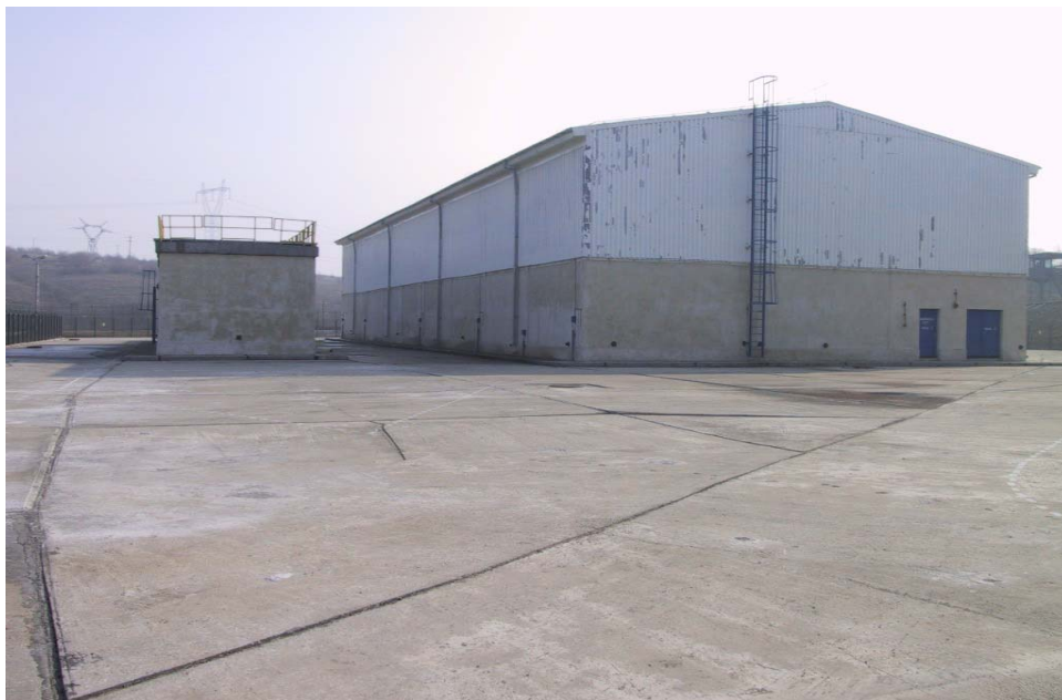
The Solid Radioactive Waste Storage Facility
